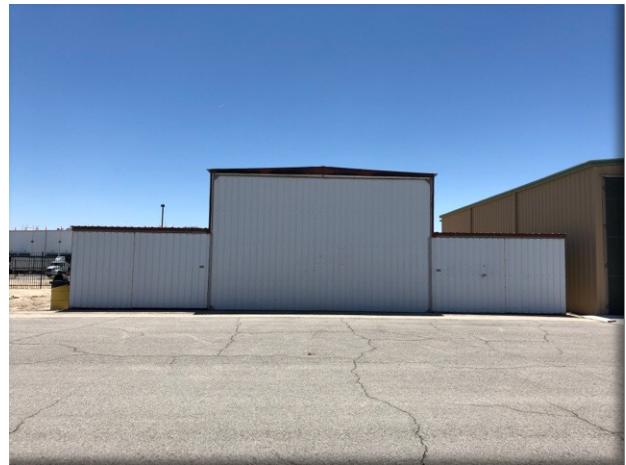
Large Portable T-Hangar 4
